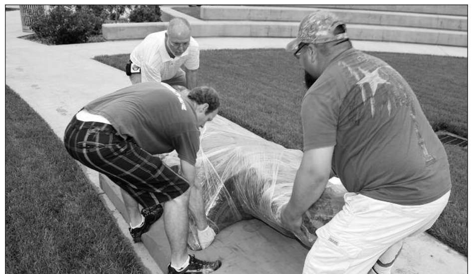
With help from Robert Cole (white shirt, facing camera), a construction superintendent at Loma Linda University, sculpture installers Ethan Johnston (left) and Jesse Cortez (right) move the weighty form of Christ onto a large piece of foam before the immense bronze sculpture was installed at the north entrance to the Centennial Complex on Friday, October 15, 2010. The pair of workmen drove the two-piece statuary installation from the Monterey Peninsula the night before.
