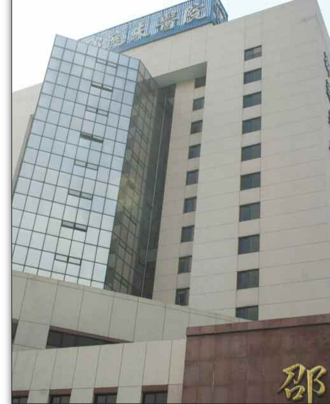
The impressive facade of Sir Run Run Shaw Hospital can be seen from miles around. The institution has become an important model of Western medicine in China. ▲
