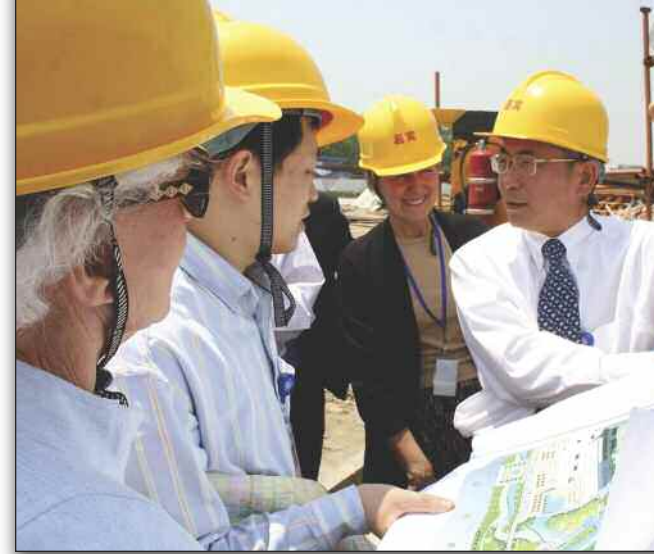
He Chao, MD (right), president of Sir Run Run Shaw Hospital, discusses construction plans with a construction official at the site of the new 1,200-bed Xiasha Hospital in Hangzhou, China. Carolyn Thompson, RN (left), a Loma Linda University Adventist Health Sciences Center councilor, and Jan Zumwalt, RN, MS, MBA (next to Dr. He), associate director of the Global Health Institute at LLU, donned hard hats for the April 29, 2009, visit. Although details are not precisely spelled out at this time, Sir Run Run Shaw Hospital is expected to assist the new facility in numerous ways. ▲
